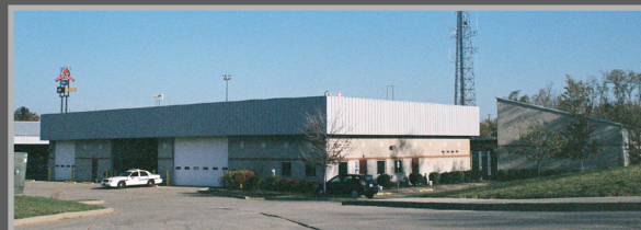
Florence Public Works - Tenured Project
