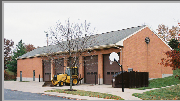
Ft. Wright Service Building - Tenured Project
